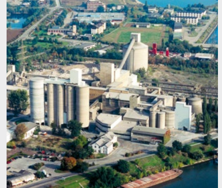
Neuwied grinding plant
