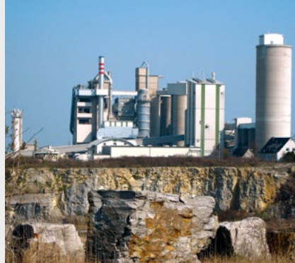
Geseke cement plant
