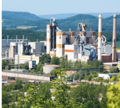
Deuna cement plant
