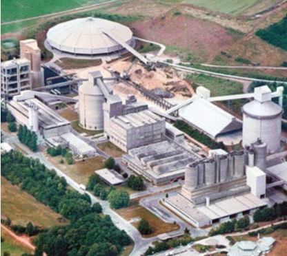
Göllheim cement plant
