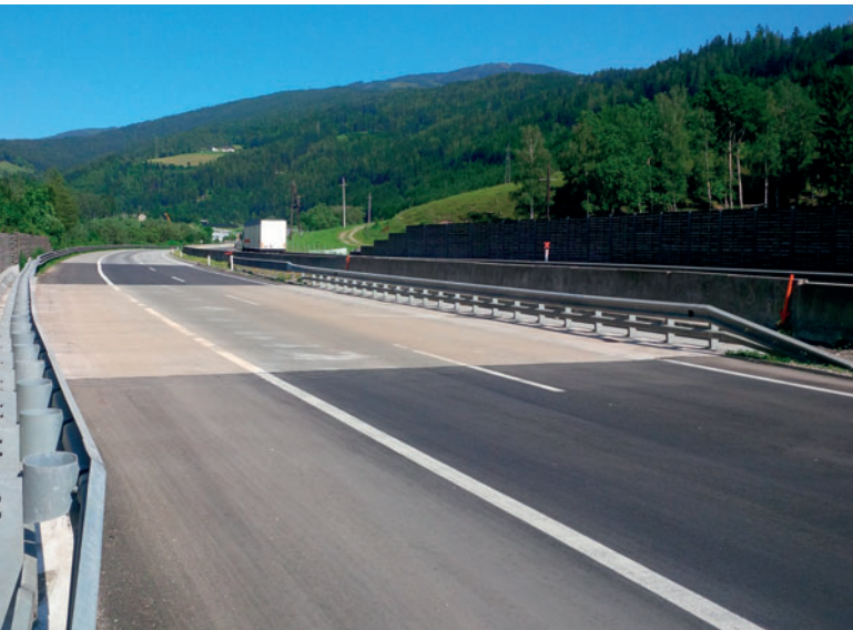
Fig. 9: Bridge strengthening (Picture: TU Graz)
