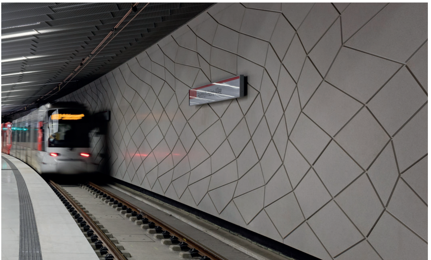
Fig. 2: Wehrhahn Underground Line Düsseldorf (Flowstone) (Picture: Joerg Hempel)
