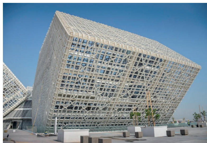
Fig. 8: Building envelope in Qatar (Picture: Ayman Badr)
